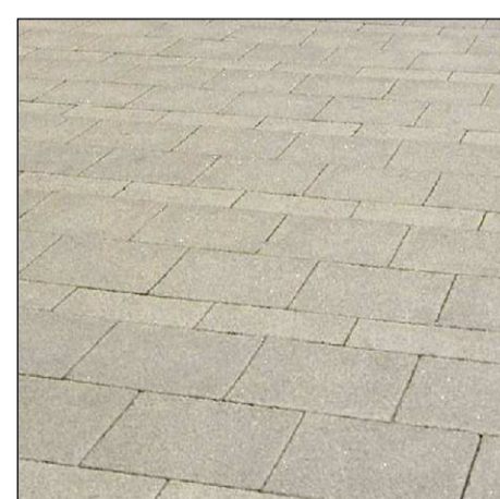
Marshall's Concrete Paving or Similar Size: 600 x 900mm Note: To adoptable standards
